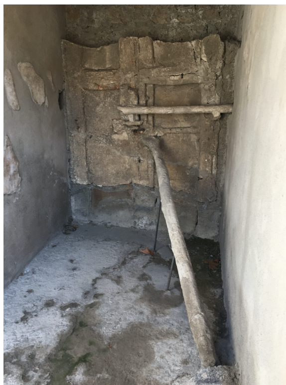
Figure 23. The entrance to the Efebo House was blocked by a pole that prevented the pumice from breaking through the door. Photo: Giacomelli and Scandone.
